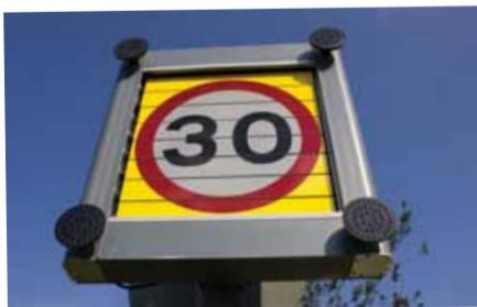
(Above) A critical part of the Heathrow project involved providing accurate info for truck drivers (Left) Variable speed zone signs are proving popular outside schools, where they can reduce speeds during term time
